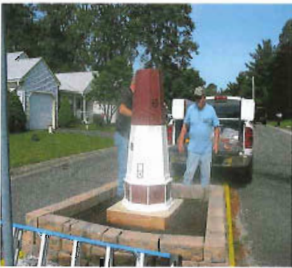
Starting to Install
